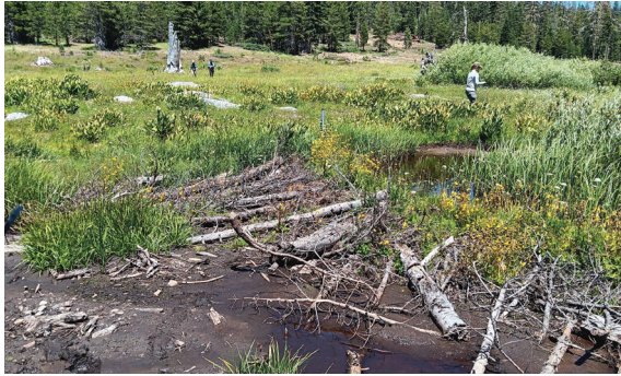
A BDA (Beaver Dam Analogue) that is part of the meadow restoration effort. These are man-made structures that mimic beaver dams to bring the water levels to the surface. [Source: Author, Eun Soo Esther Shin]
